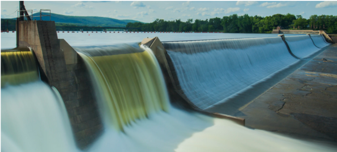
Holyoke Dam: Powering Hazen Paper with Hydropower
